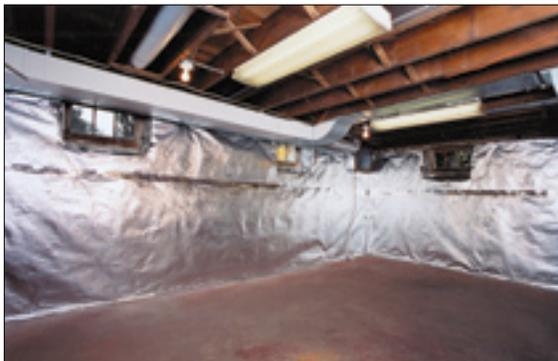
Using the ThermalDry® Wall System to cover your basement walls helps to insulate your home, reflecting over 90% of the heat back in. Use when you plan to conventionally finish your basement.
